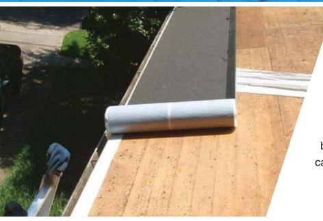
Techno Phase membranes are designed for use where direct torching to the roof deck is to be avoided because of a risk of burning.
