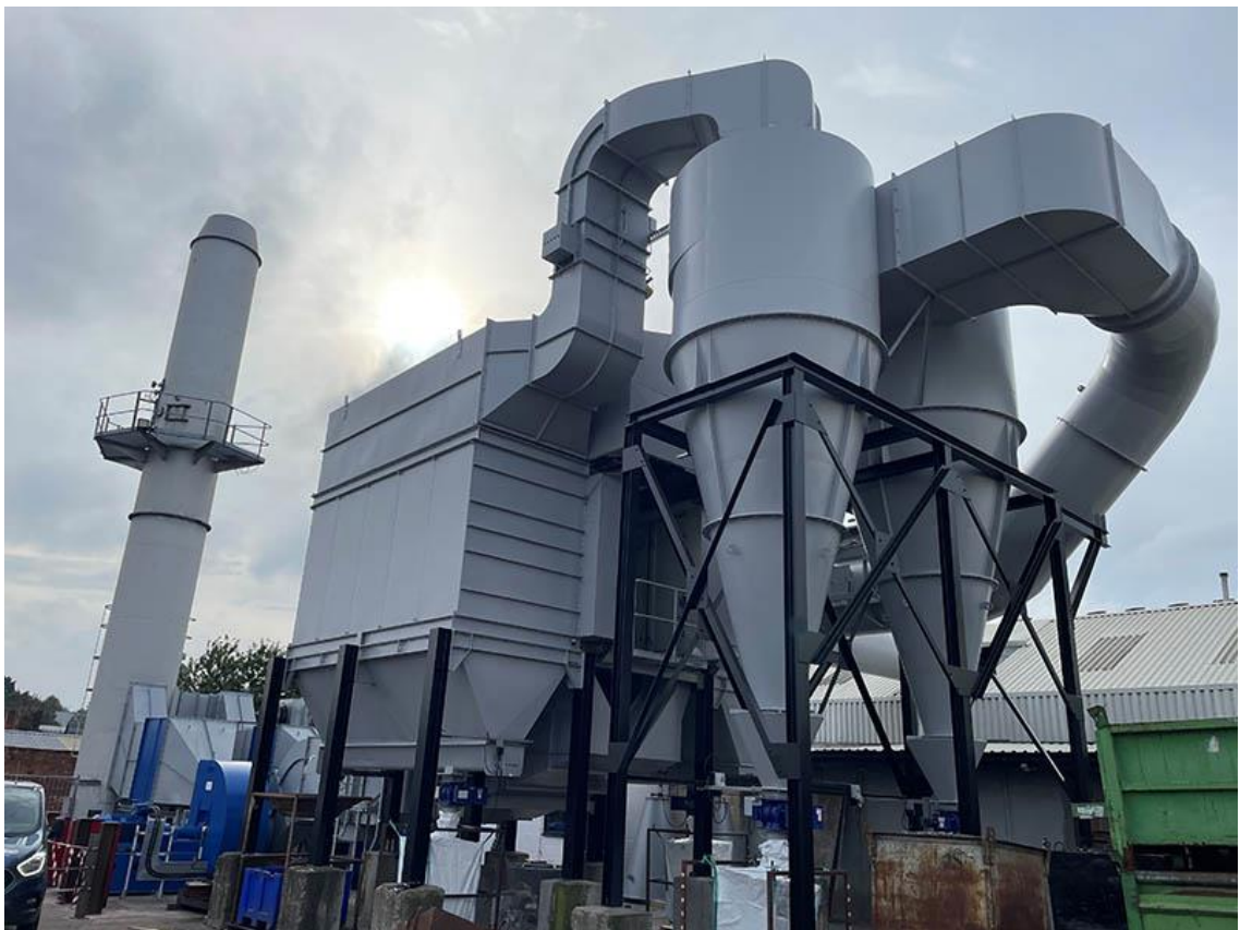
Foundry Flue Gas Treatment System Upgrade - Birmingham
